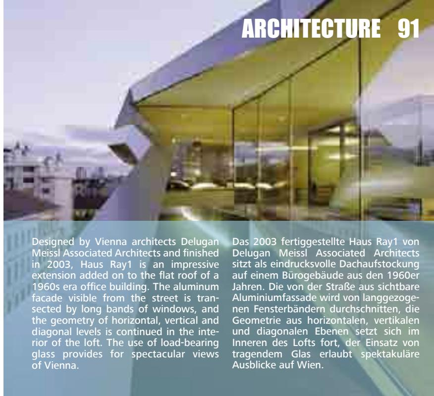
Designed by Vienna architects Delugan Meissl Associated Architects and finished in 2003, Haus Ray1 is an impressive extension added on to the flat roof of a 1960s era office building. The aluminum facade visible from the street is transected by long bands of windows, and the geometry of horizontal, vertical and diagonal levels is continued in the interior of the loft. The use of load-bearing glass provides for spectacular views of Vienna.
